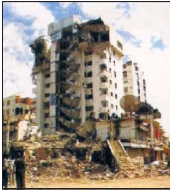
Fig. 3.3a: Destruction caused by an Earthquake at Bhuj
