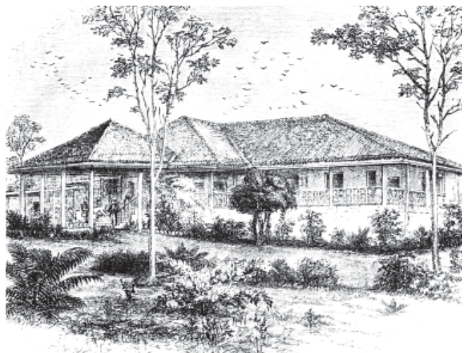
Fig. 12.23 A bungalow in Bombay, nineteenth century
