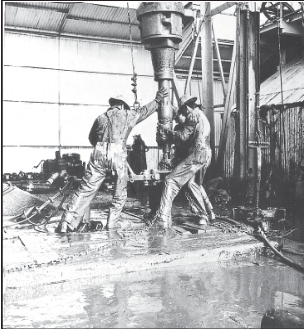
Fig. 5.18: Oil drilling operation in the Gulf of Mexico
