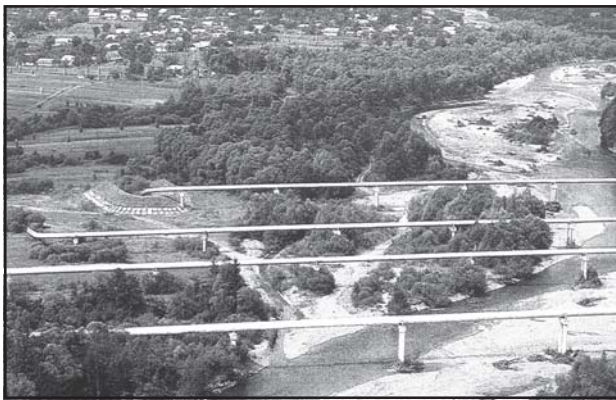
Fig. 8.17: Pipelines transporting natural gas in Ukraine
